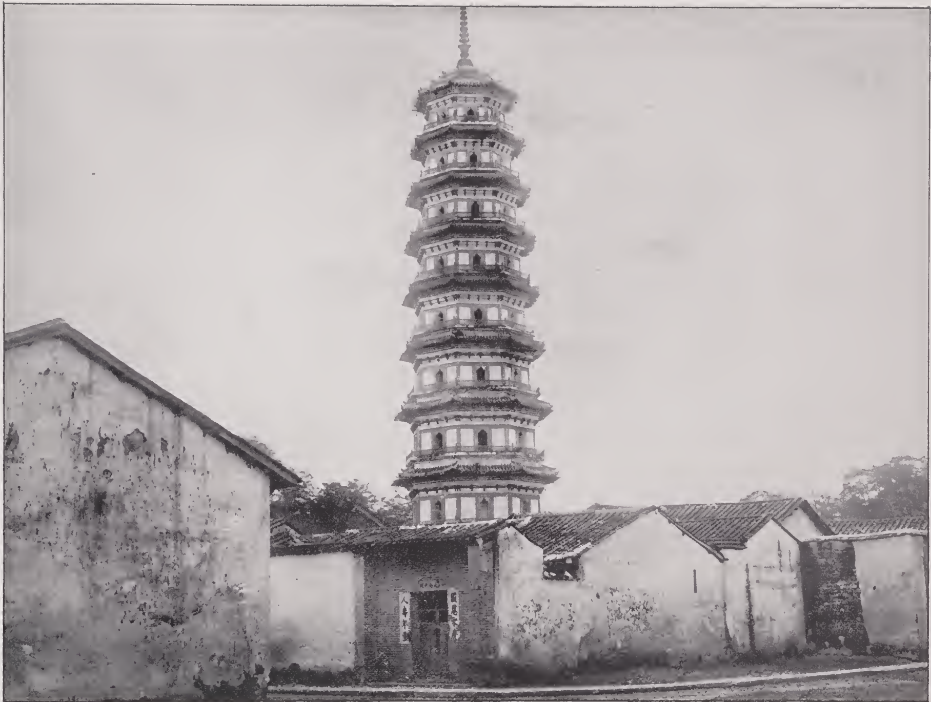
NINE STORY PAGODA, CANTON, CHINA.—This is one of the most celebrated of this class of buildings in China. It is an octagonal pagoda, of nine stories, 170 feet in height and was first erected thirteen centuries ago. Brick, covered with marble or glazed tile, was the material used in construction. Each story is reduced in width and has a gallery round it. The roofs are hollow and sagging. They project a great deal, the corners being turned up sharply. In these corners, light bells are suspended, which make a constant ringing when the wind blows.
